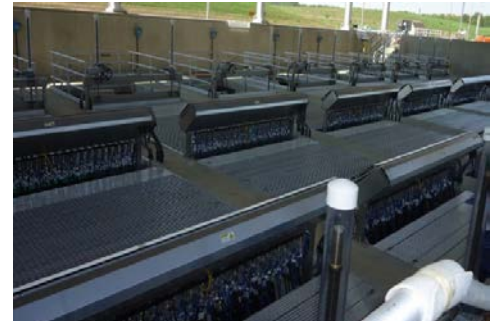
Figure 2: UV disinfection System in Belmont Waste Water Treatment Plant
