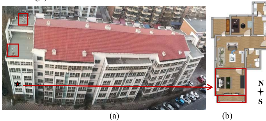
132 133 134 Fig. 1. (a) Apartment building in Tianjin, China, with weather stations on the roof as indicated by the 135 two red boxes and (b) floor plan of the two-bedroom apartment
