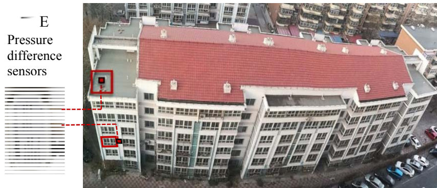
184 185 Fig. 3. Schematic of pressure measurement positions near the window and the reference position at 186 the weather station 187
