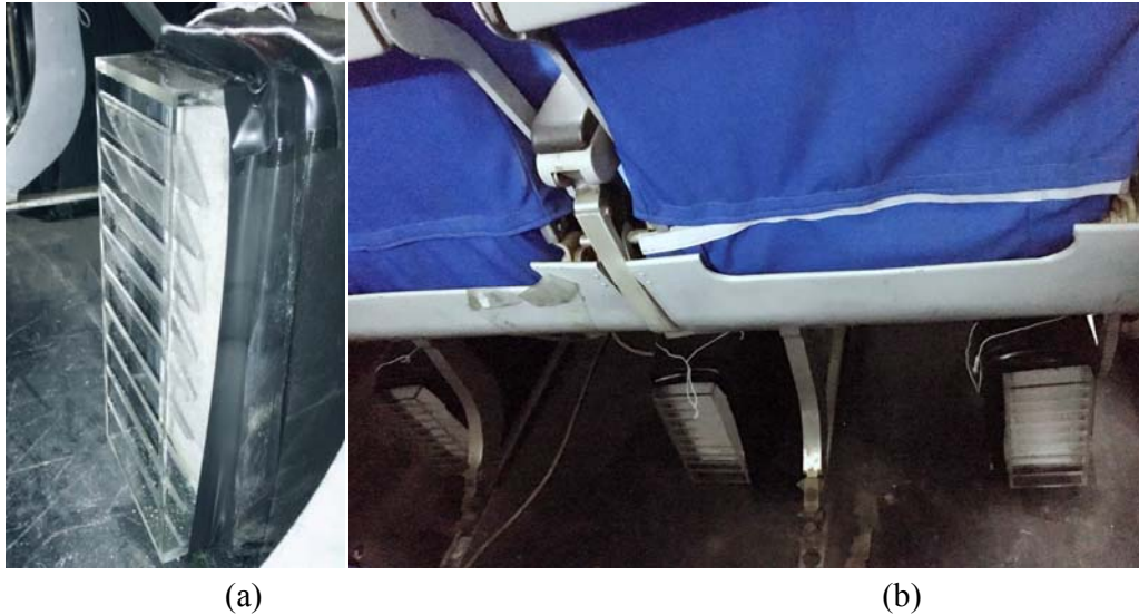
Figure 5. (a) A close-up view of a diffuser and (b) the diffusers installed under the seats.
