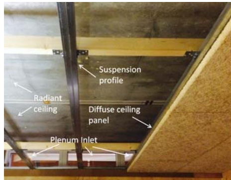
Fig.4. Diffuse ceiling panels and radiant ceiling
