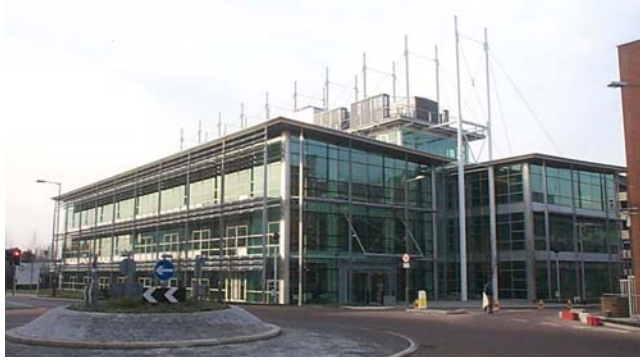
Fig. 4. BP Sunbury Building A
