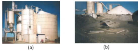
(B) Photographs of the thermal ratcheting failure of a bin containing 9000 tons of fly ash. Photographs from Dogangun et al. [12].
