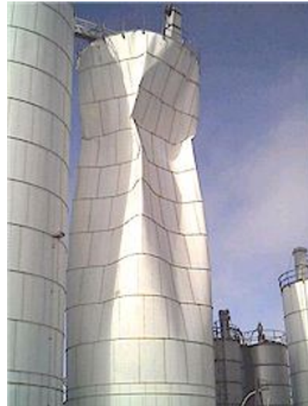
(B) A photograph of a silo with buckled walls caused by pressure differences.
