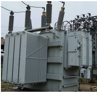
LTC transformer (substation regulator)
