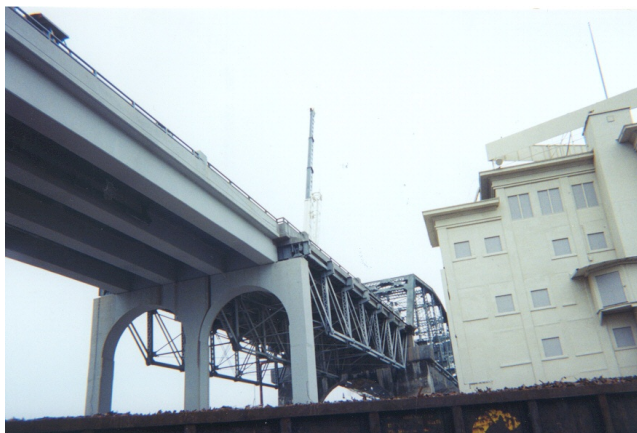
Figure 6: View of approach superstructure
