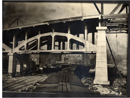
Figure 3: Concrete Truss under construction
