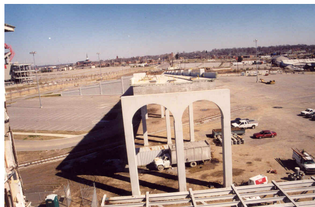
Figure 5: View of approach piers
