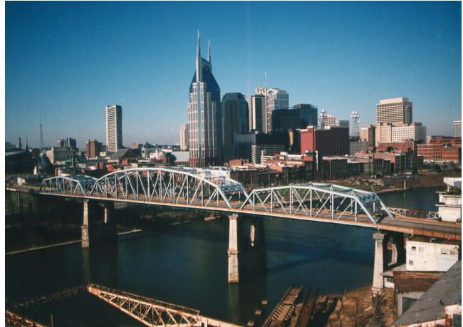
Figure 1: View Looking North
