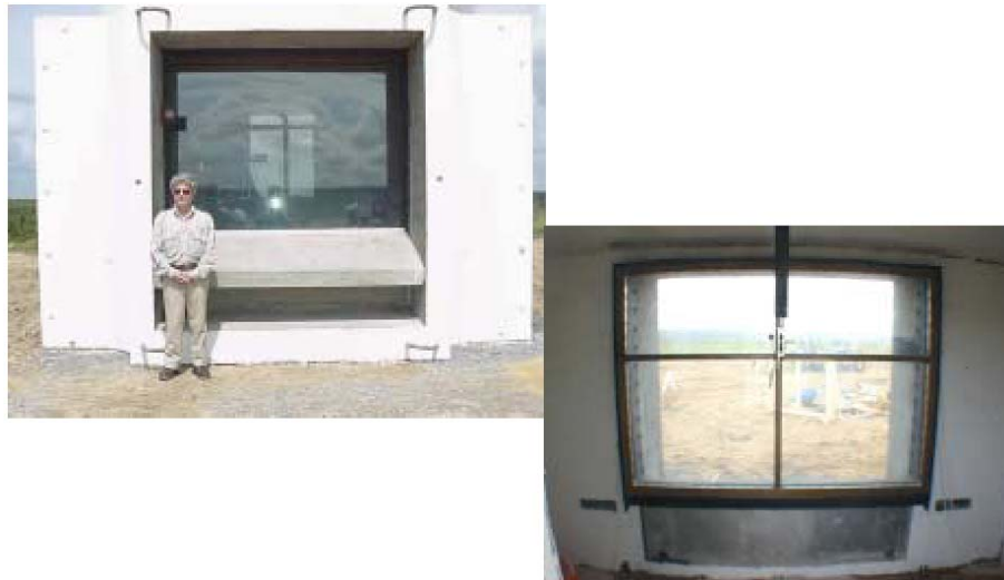
Figure 4: Installed Muntin System 9
