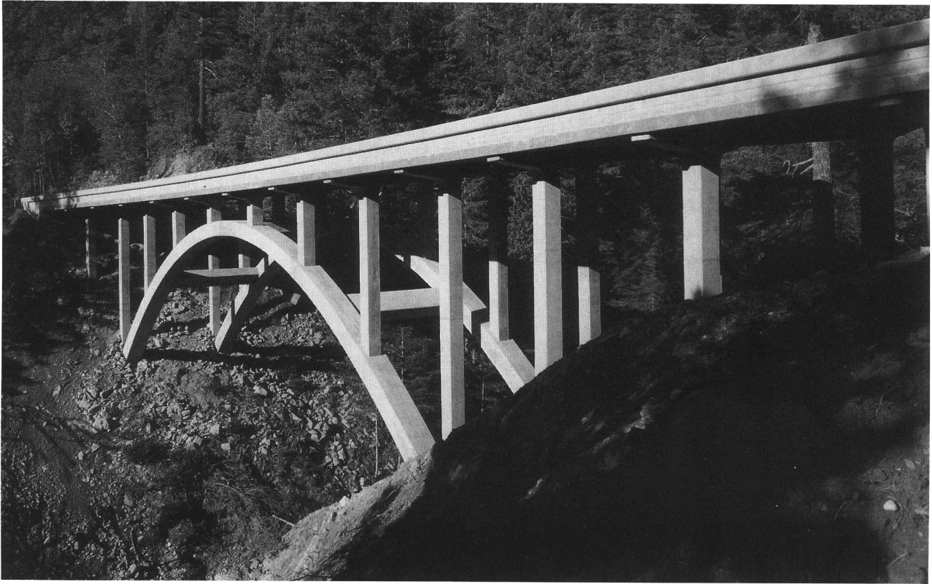
Myrtle Creek Bridge in California used precast elements
