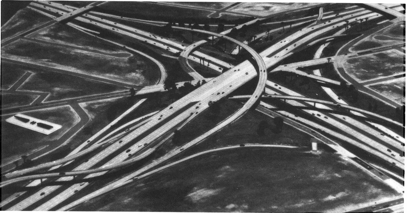
Complex highway interchange in California with fifteen bridge structures
