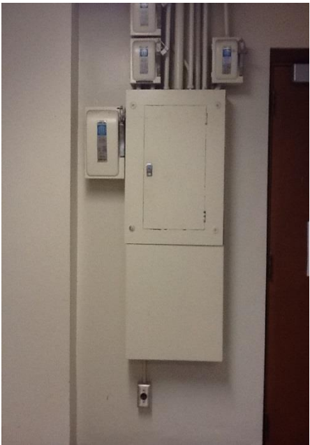
Electrical Panel with tapped disconnects
