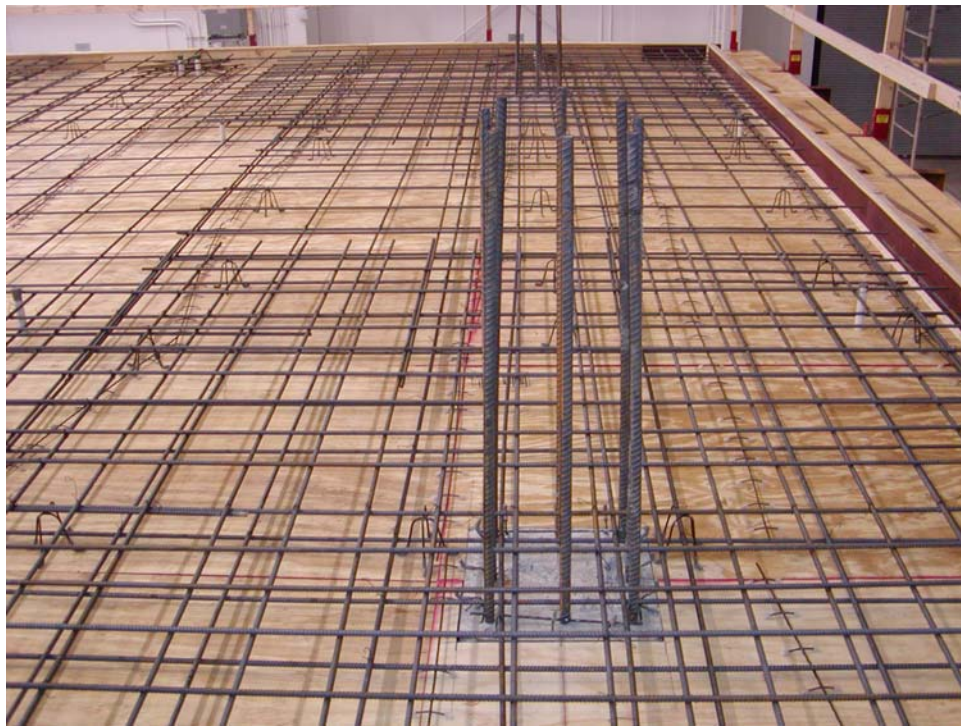
Figure A-14 Slab Reinforcement
