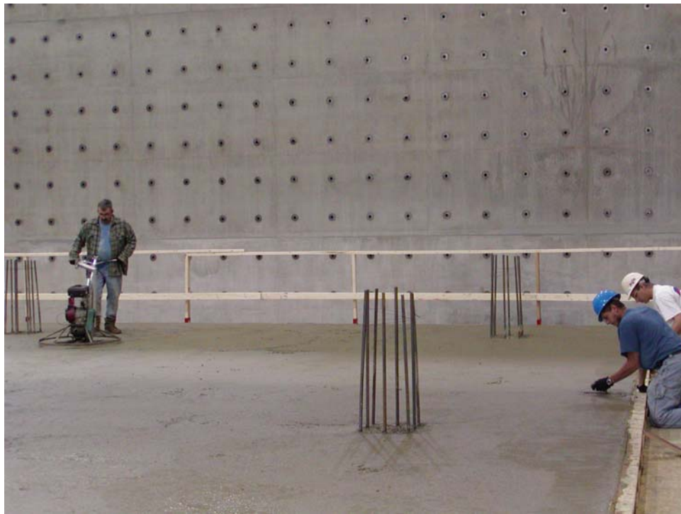
Figure A-16 Concrete Finishing
