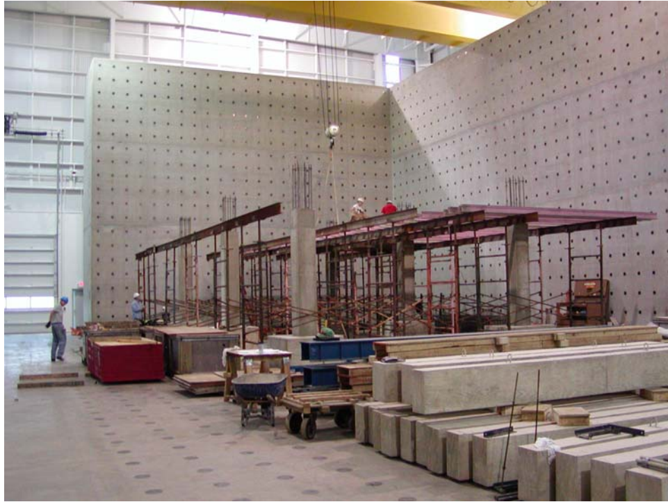
Figure A-13 Level 1 Slab Shoring
