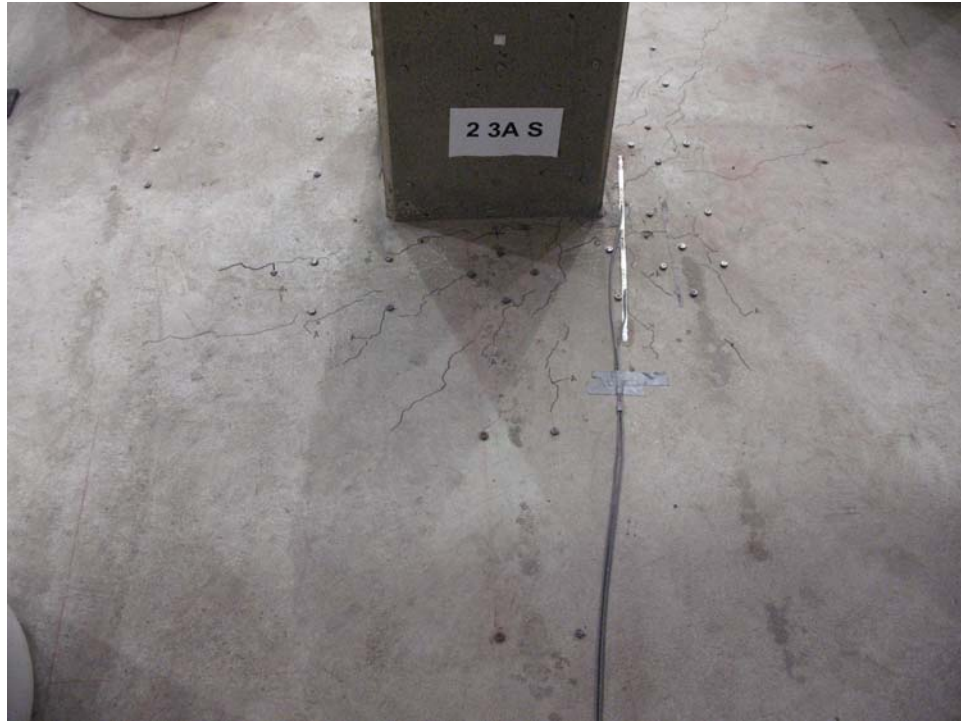
Figure 3-76 Level 2 Column 3A South Initial Cracks
