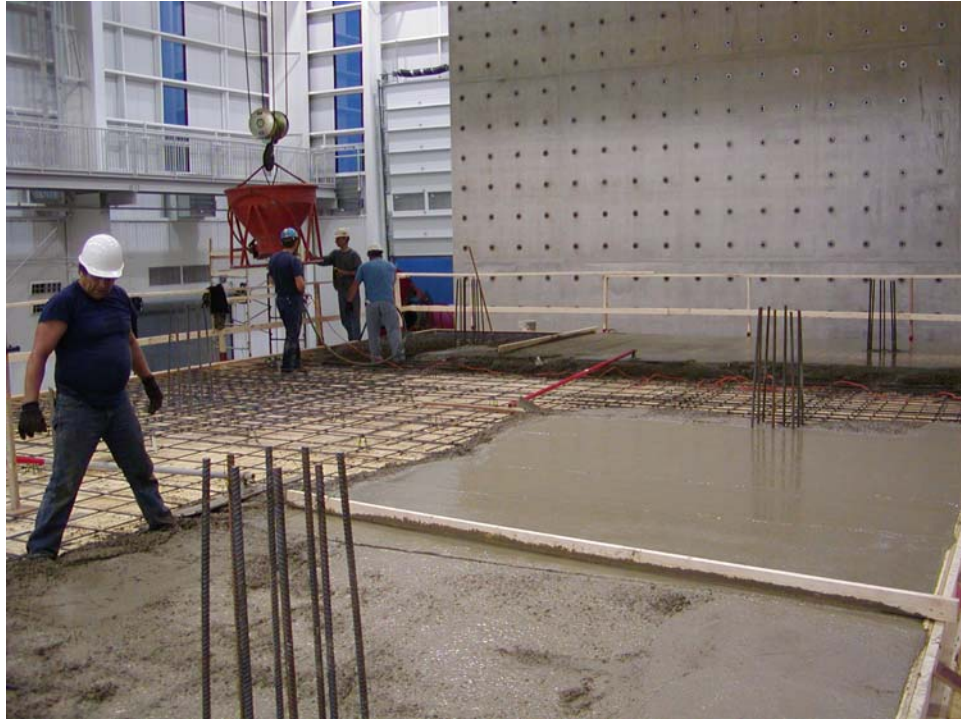
Figure A-15 Concrete Placement
