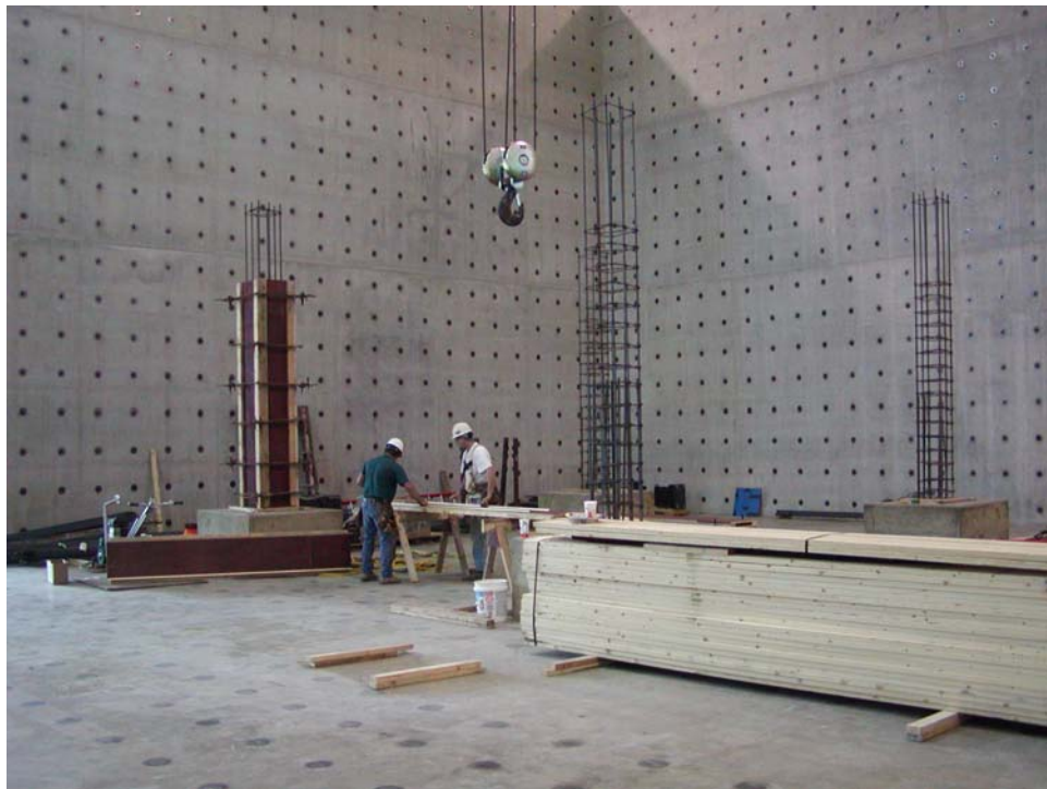
Figure A-12 Level 1 Column Cage and Forms
