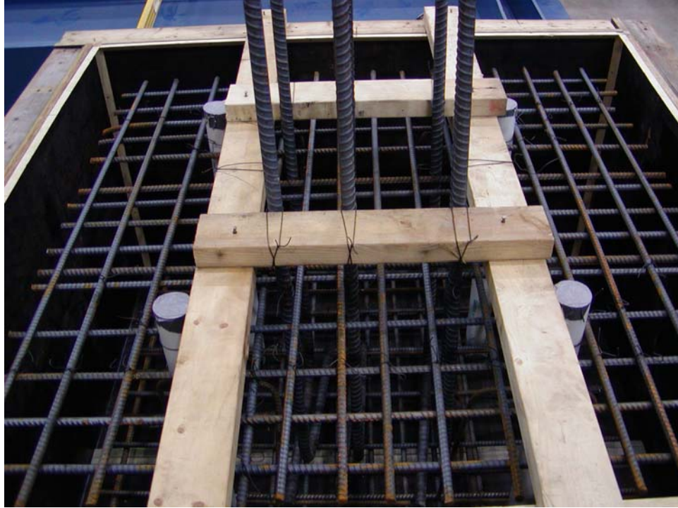
Figure A-11 Footing Reinforcement
