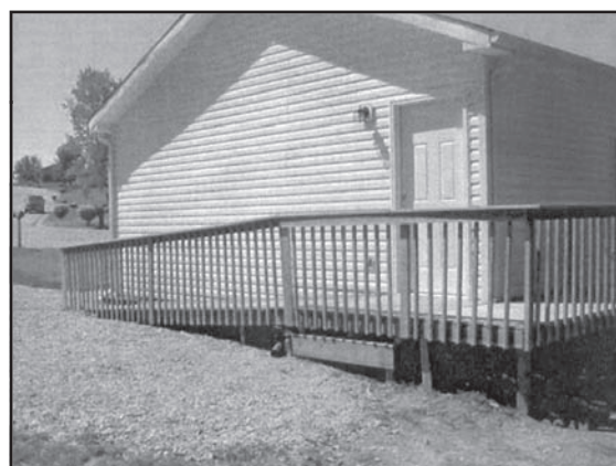
West Washington's ramp and deck extension
