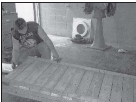
A West Washington FFA member constructs a wheelchair-accessible ramp
