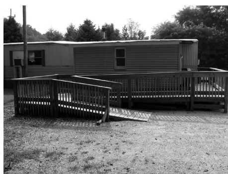
Figure 1: Modular ramp at 1 st location
