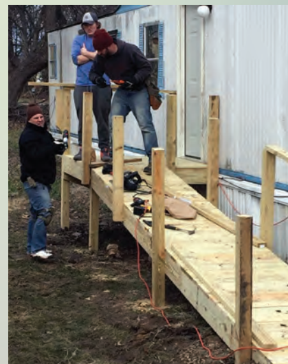
Members of the Embassy Men group build a wheelchair-accessible ramp
