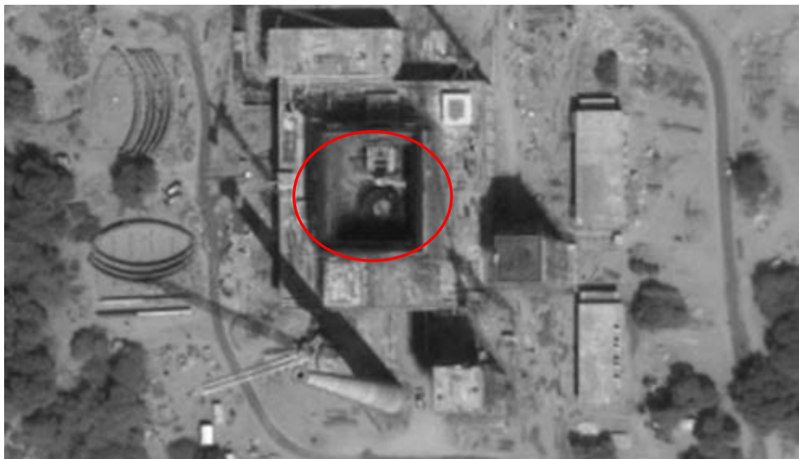
Pléiades image over the same area, dated March, 28 th 2012: vessel is seen inside the reactor building © CNES – Distribution Astrium Services / Spot Image
