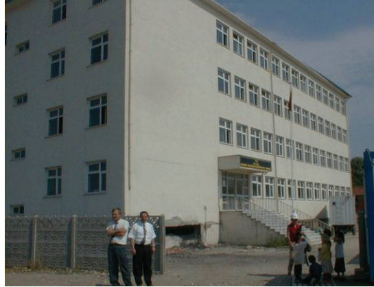
Figure 12. A four-story dual-system building in Düzce (Building D02).
