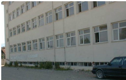
Figure13. View of the captive exterior columns in the basement of Building D02 from outside and inside. The columns are captive in their weak axis.
