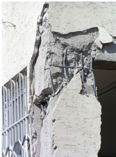
Figure 15. Typical column end reinforcement detailing exposed in Building C14-01.
