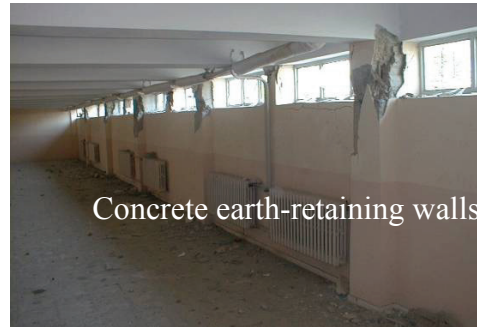
Figure13. View of the captive exterior columns in the basement of Building D02 from outside and inside. The columns are captive in their weak axis.
