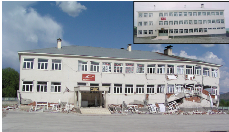
Figure 8. Building C13-08 before (small photo) and after (big photo) the 2003 Bingöl earthquake. The first story is completely collapsed during the earthquake. The captive columns in the ground floor were shown at the right end of the school (small photo).
