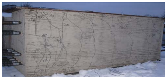
Fig. 26: Concrete crack map after test completion
