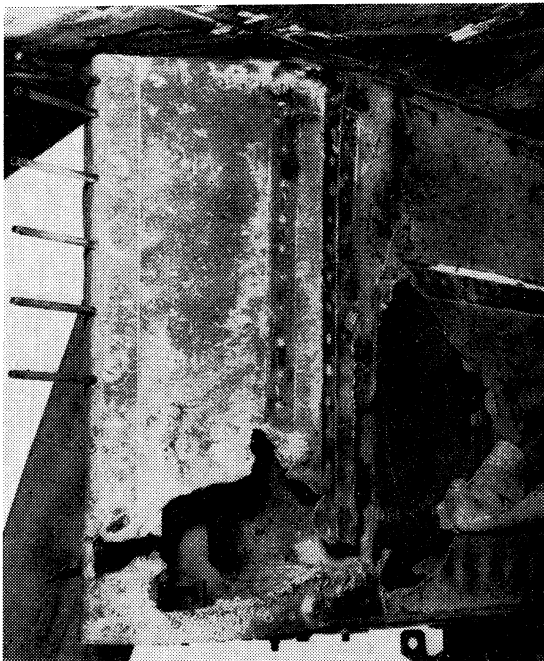
Fig. 1.7. Side view of ventral fin showing damage due to shock impingement. (Photo courtesy of NASA.)
