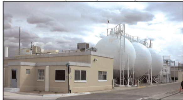
The Engineering Sciences Experimental Facility houses Sandia's experimental aerodynamics wind tunnels. The HAC is the third sphere (furthest to the right) of the vacuum system used for HWT operations.
