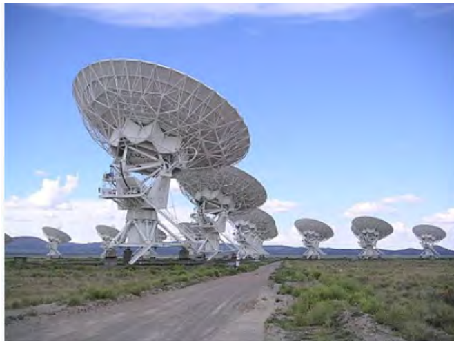
Figure 24.3: Picture of the Very Large Array in New Mexico, USA (courtesy of [168]). The low loss of the circular waveguide gives good SNR (signal-to-noise ratio) according to the fluctuation dissipation theorem, which makes the system good for detecting weak radio astronomy signals from outer space.
