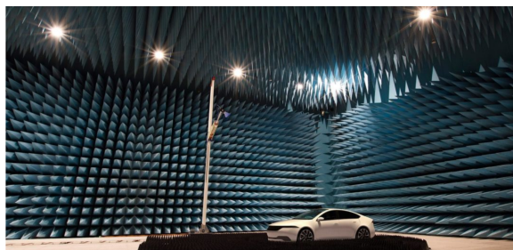
Figure 37.5: An anechoic chamber for radio frequency. In such an electromagnetically quiet chamber, interference from other RF equipment is minimized (courtesy of Panasonic).
