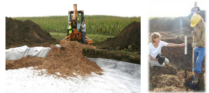
Filled 3-ft high woodchips; 4 PVC wells
