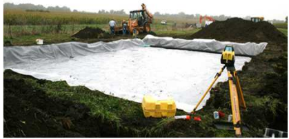
Subsurface trench lined with plastic
