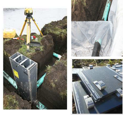
Drainage control structures
