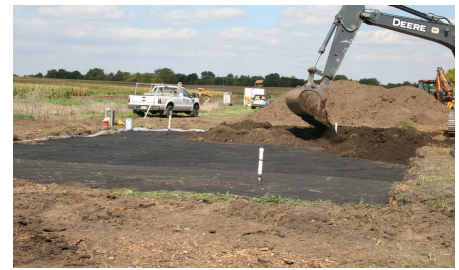
Topped with geotextile and 1-ft topsoil
