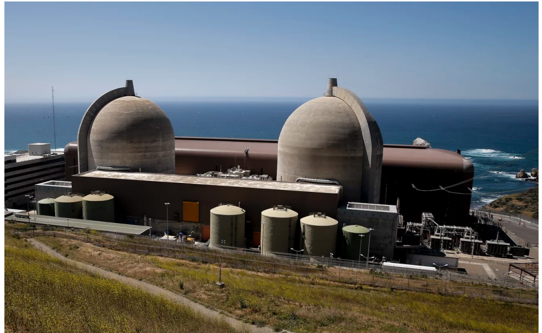
Diablo Canyon Nuclear Power Plant in California
