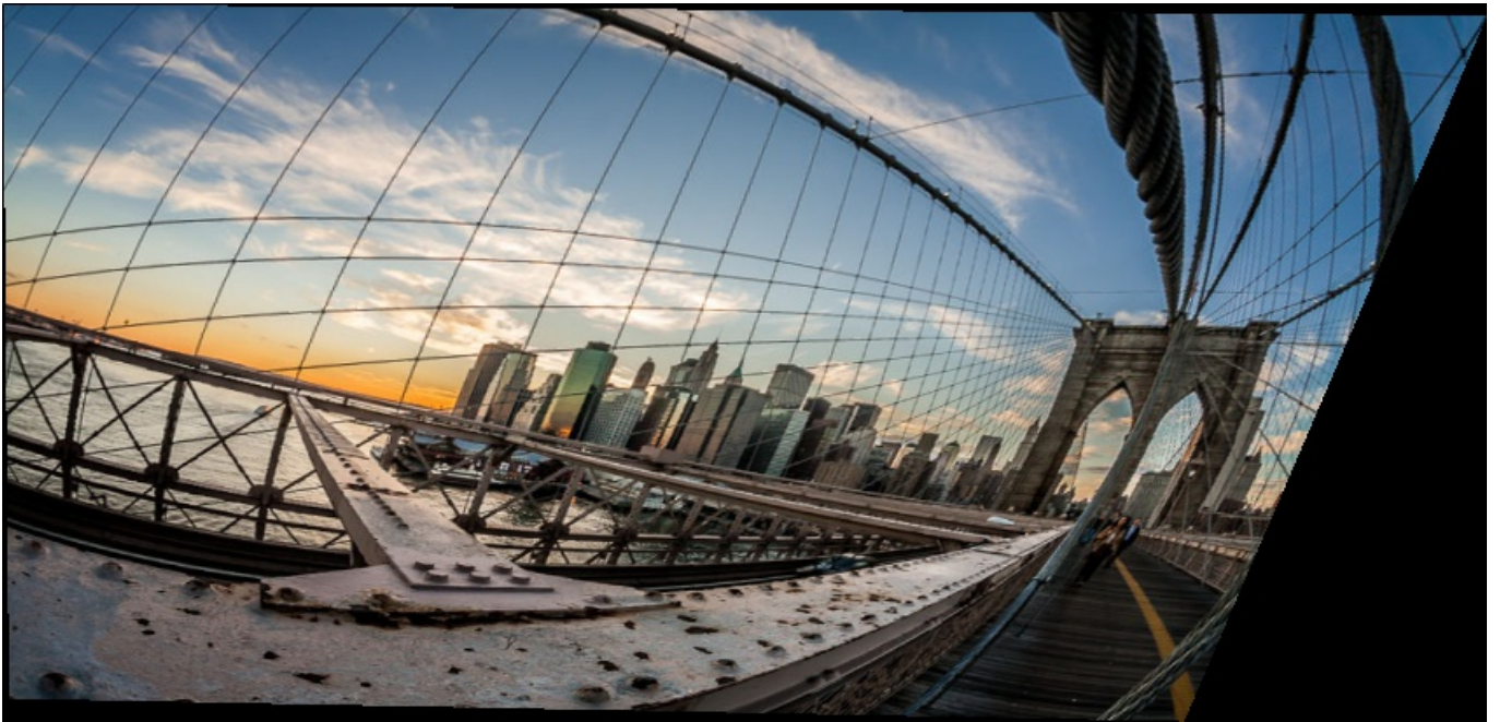
Figure 14: Results obtained using Method 2: Two Step Method :- Removing Affine Distortion as well as Projective Distortion
