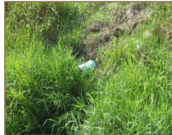
Tile drain outlet
