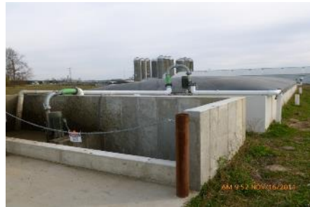
Plug flow system (1000 m 3 )
