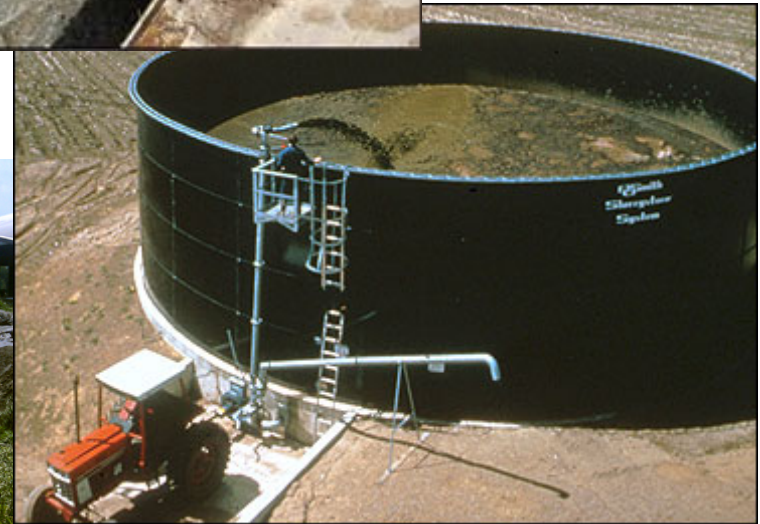
Above ground storage tank
