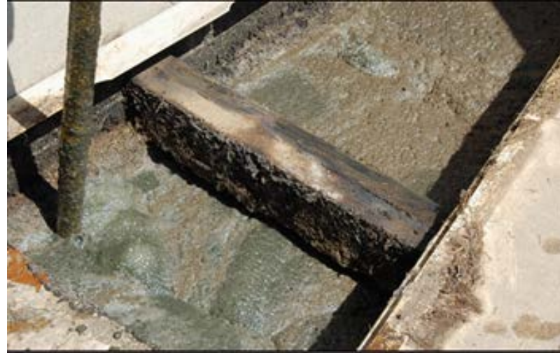
Below ground pit
