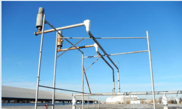
Includes a 5.0 million-gallon digester
