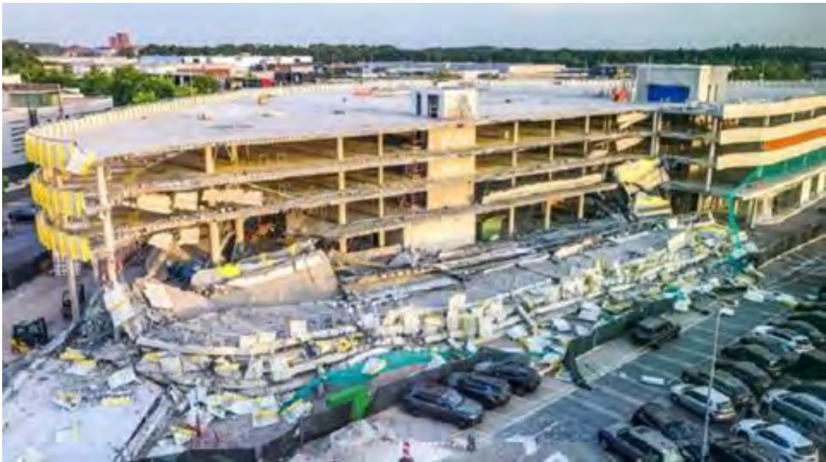
Fig. 1.1. The Eindhoven parking garage collapse in 2017 [1].
