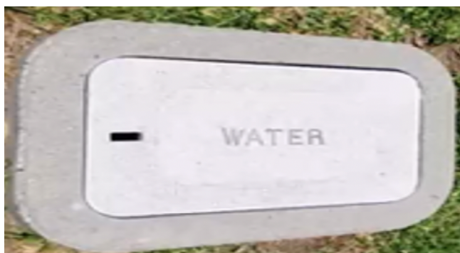
Concrete Meter Boxes Credit: Paradise Irrigation District
