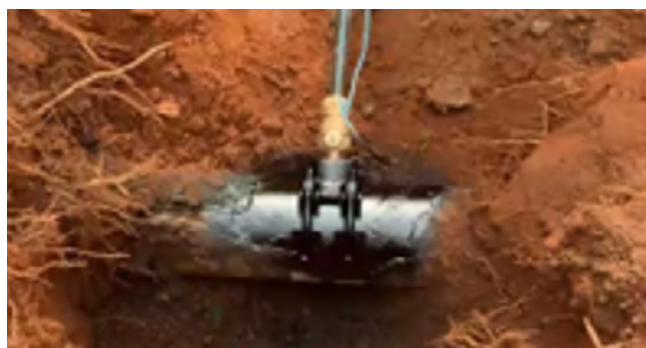
Service Line Replacement Credit: Paradise Irrigation District
