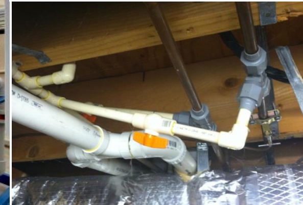
Copper pipe to cPVC pipe
