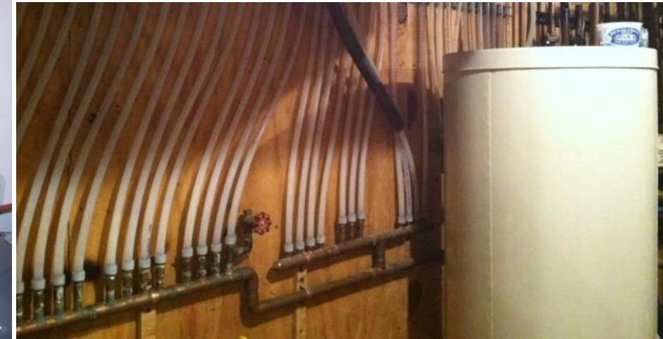
Copper pipe to cPVC pipe
