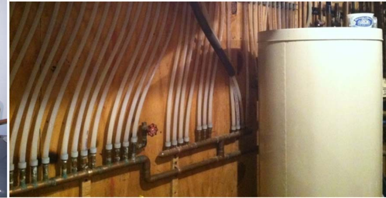
Copper pipe to cPVC pipe
