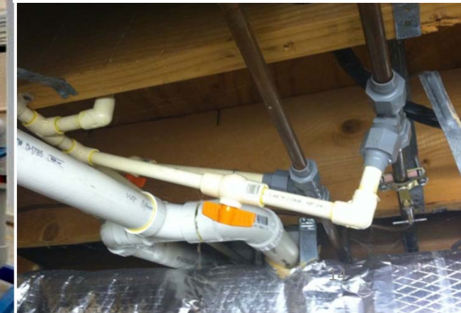
Copper pipe to cPVC pipe
