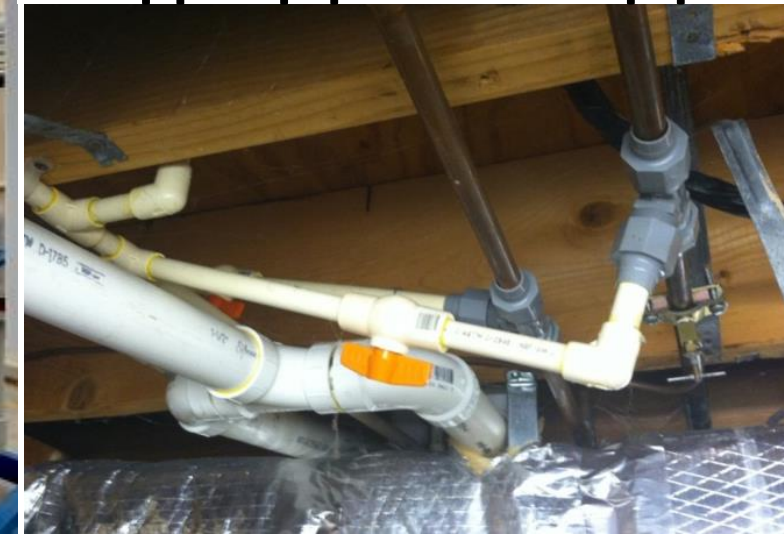
Copper pipe to cPVC pipe
