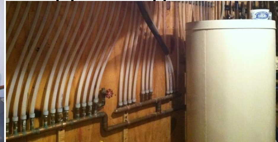
Copper pipe to cPVC pipe
