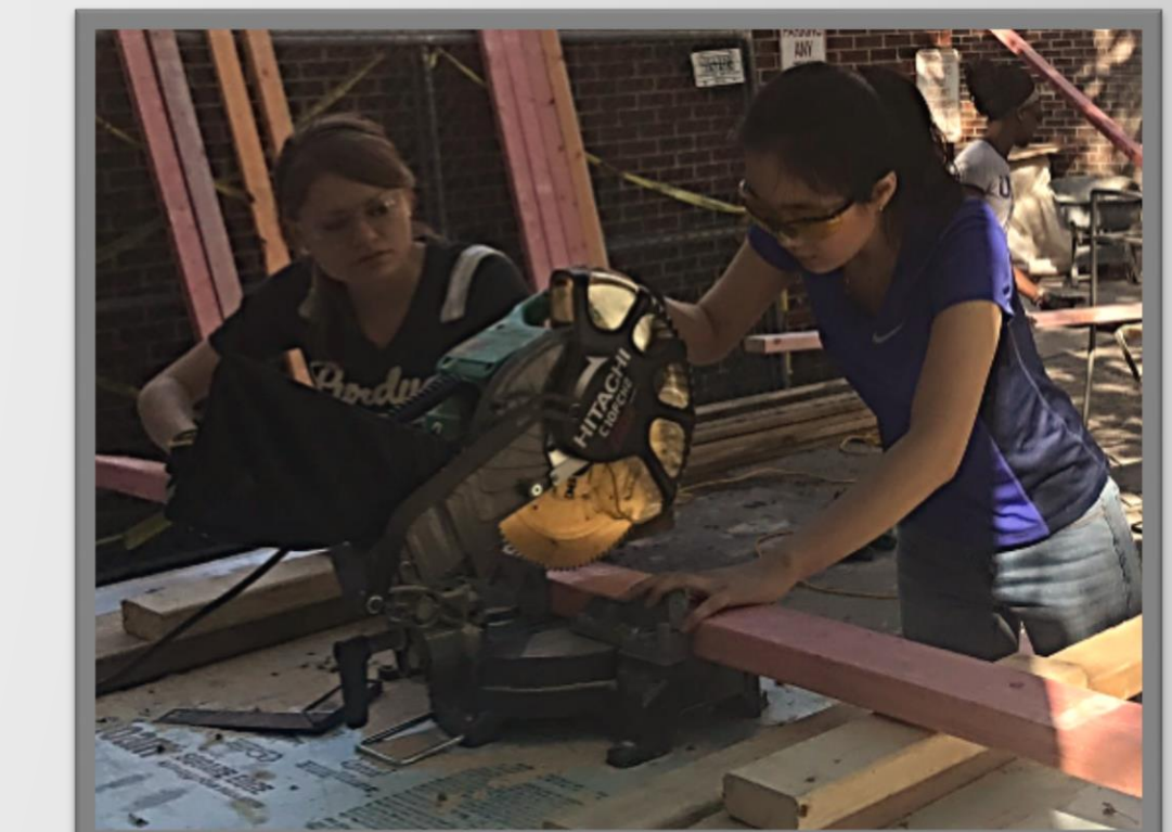
Figure 3: Pilot-scale plumbing rig construction underway
