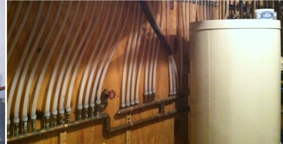
Copper pipe to cPVC pipe
