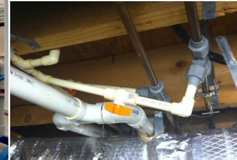
Copper pipe to cPVC pipe
