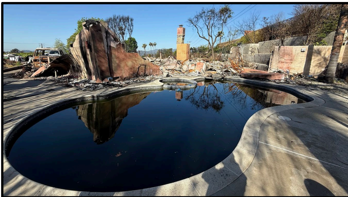
Pools were sometimes impacted by fire debris, but not all properties had a pool.
