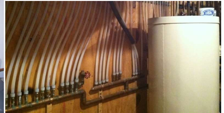
Copper pipe to cPVC pipe
