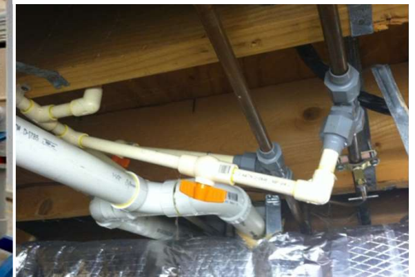
Copper pipe to cPVC pipe
