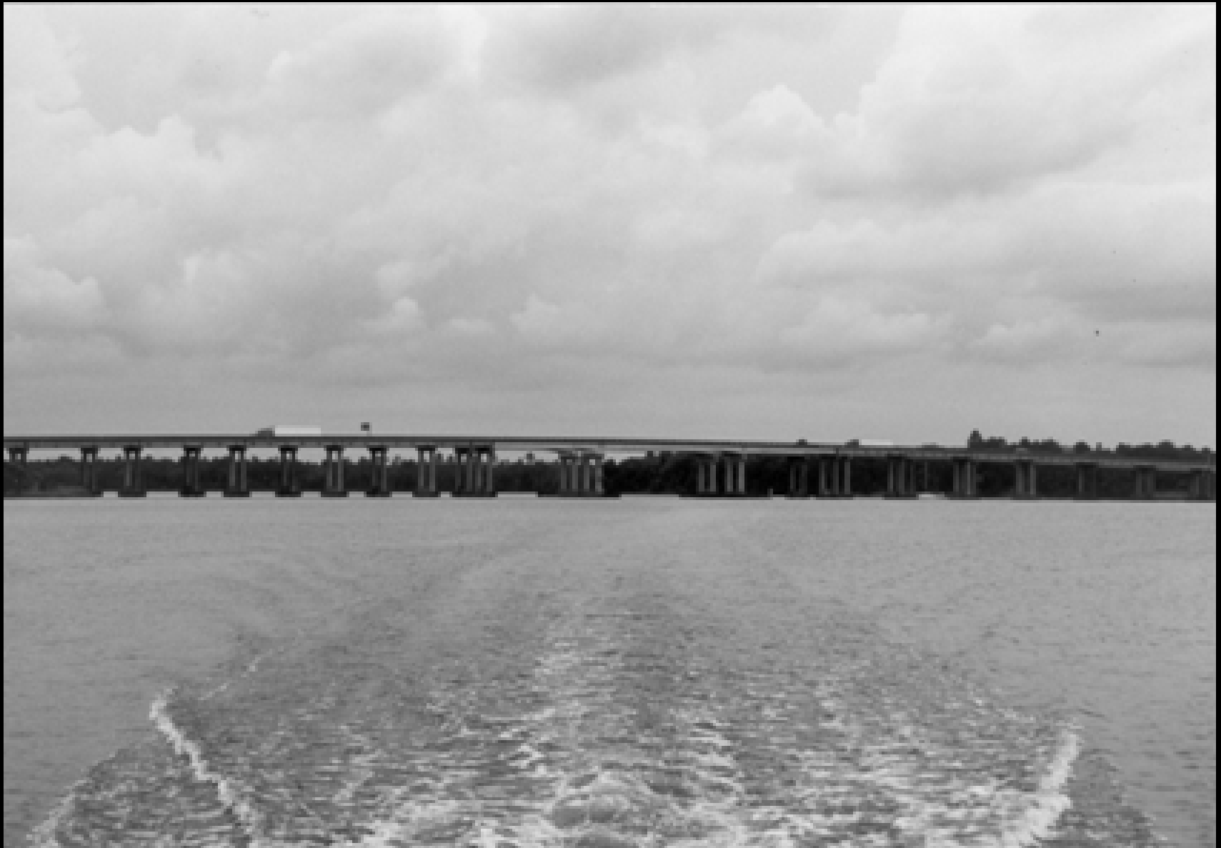
BLACKWATER RIVER BRIDGE looking SOUTH
