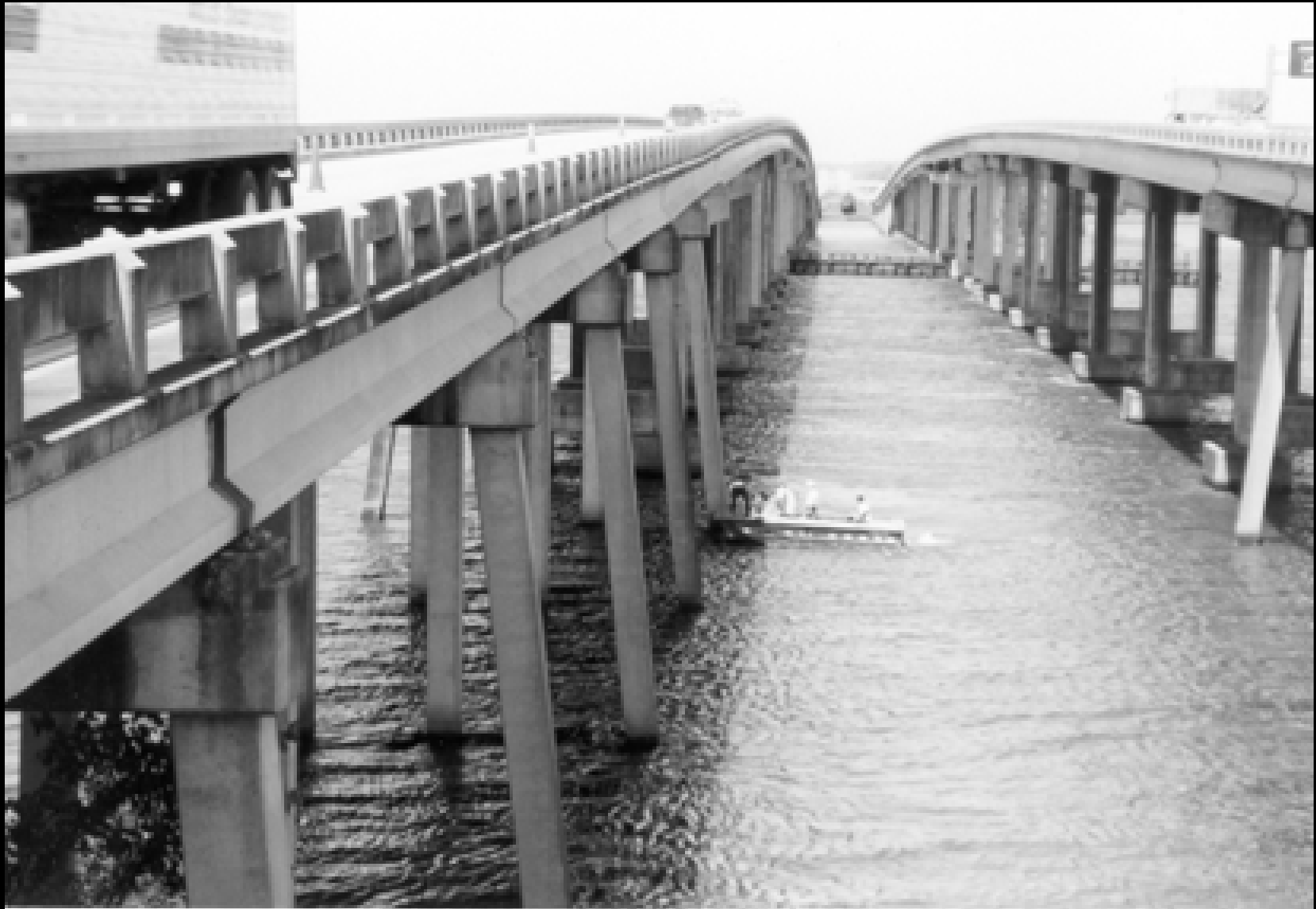
BLACKWATER RIVER BRIDGE looking WEST
