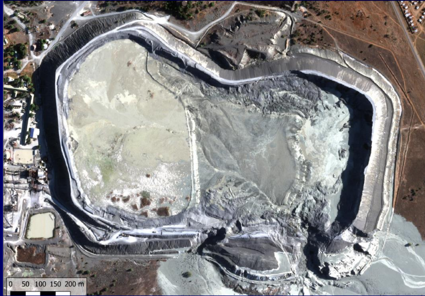
Jagersfontein Tailings Dam Failure South Africa, 11 September 2022
