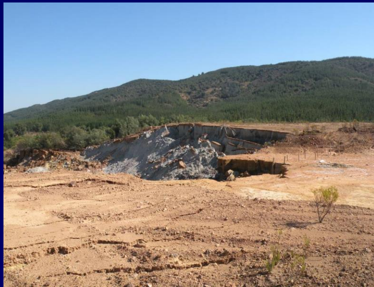
View across scarp
