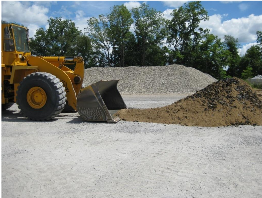
Loader bucket used to thoroughly mix shredded tires and sand
