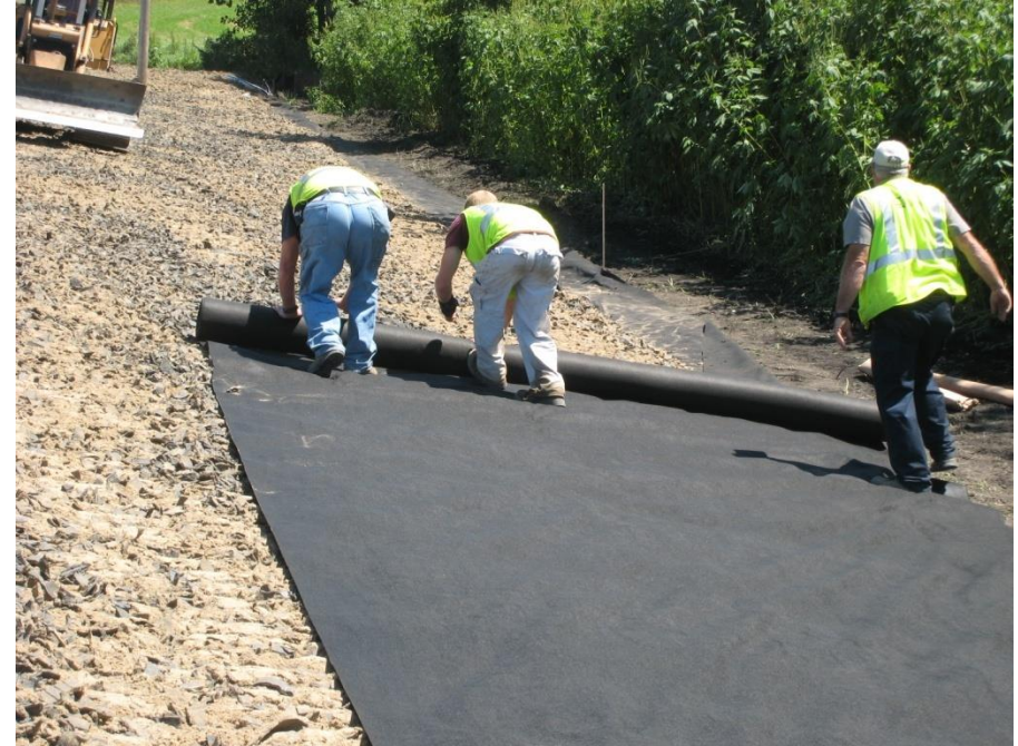
Finally, encasing the side slopes with geotextile
