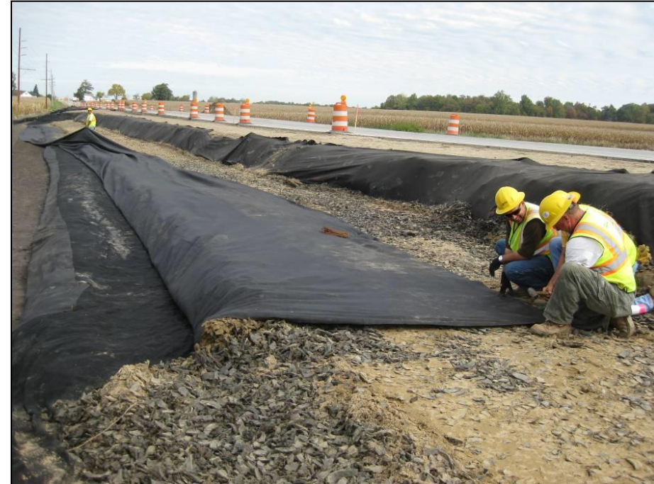
Geotextile wrapped around compacted lift of mixture
