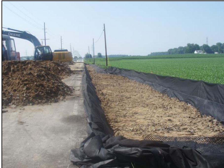
Mixture awaiting wrapping of geotextile
