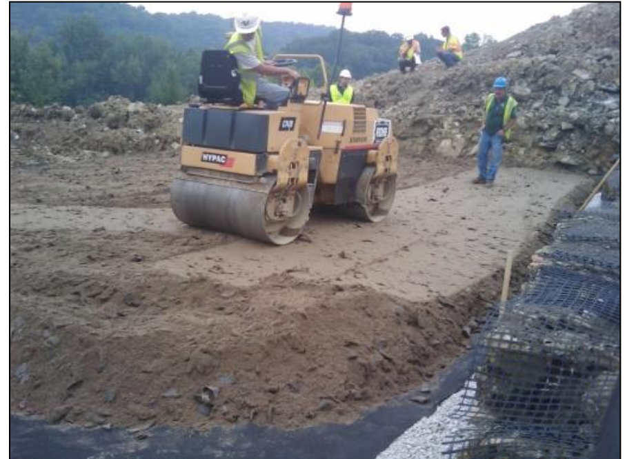
Hauling and compacting the mixture (10 ton roller, lifts of 12 inches)
