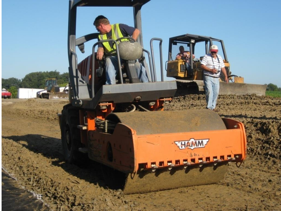
Mixture being compacted using 5 T smooth-drum roller
