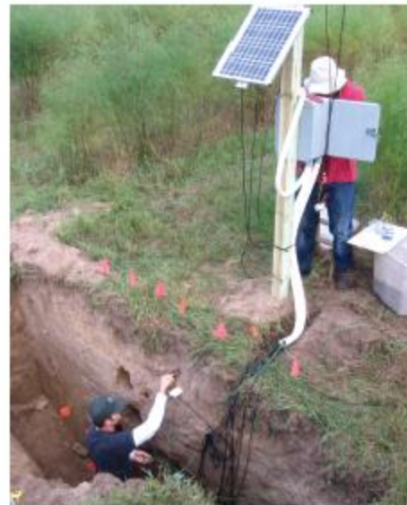
Figure 5. Photograph showing installation of subsurface instruments into trench face.
