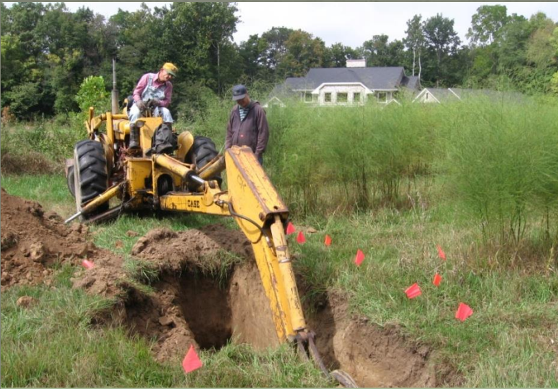
Trenches excavated to 2 m/6 ft depth at six locations across the State
