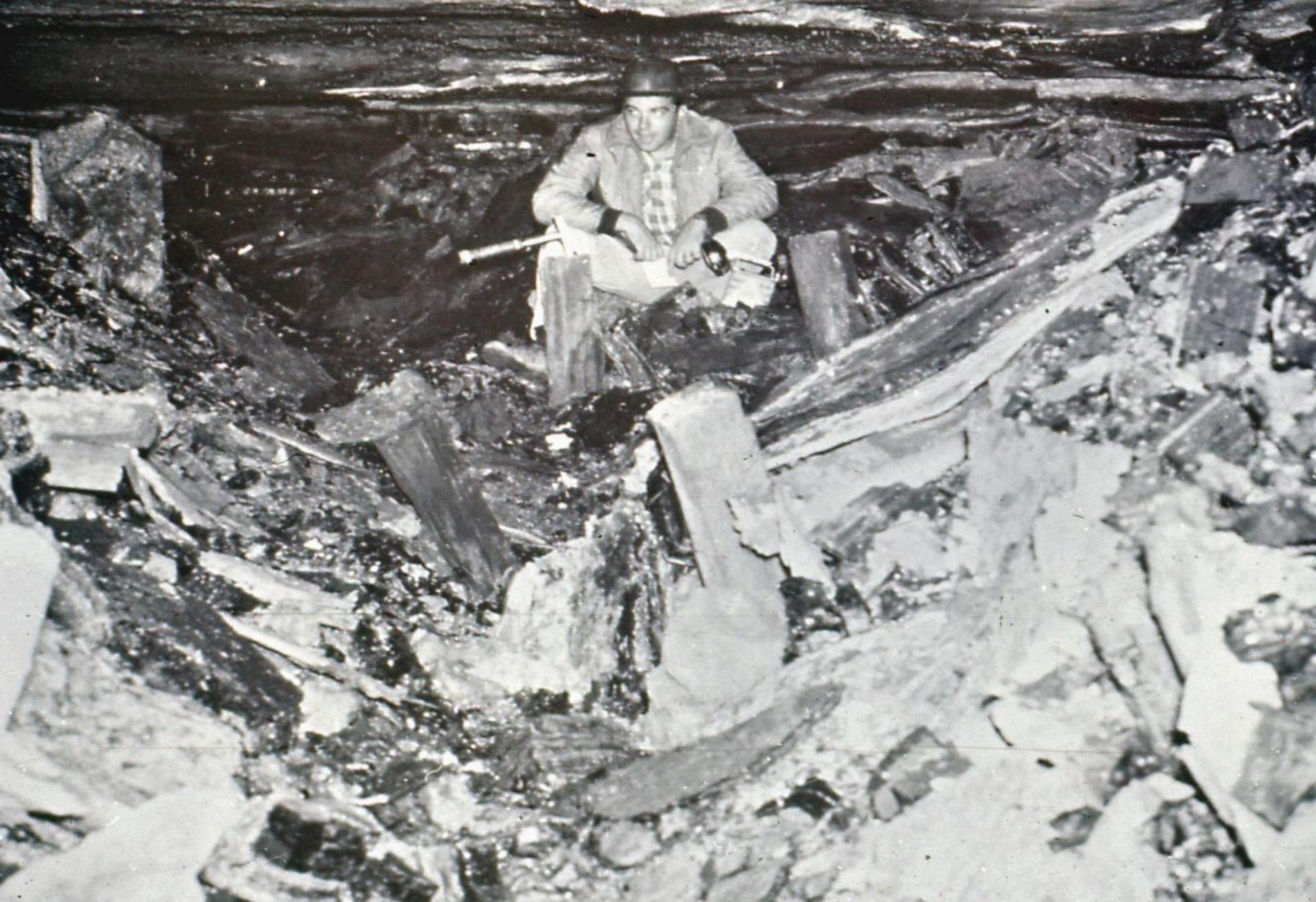
ABANDONED MINE IN PITTSBURGH COAL
