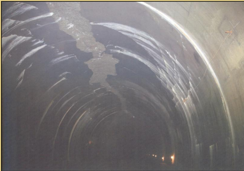
Longxi Tunnel, after 2008 Wenchuan earthquake, China (courtesy of Dr. H. Yu)
