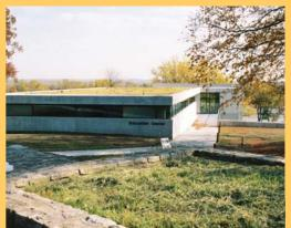
LEED<sup>®</sup> Gold Rating with green roof, radiant heating and cooling, passive solar heating and natural ventilation.
