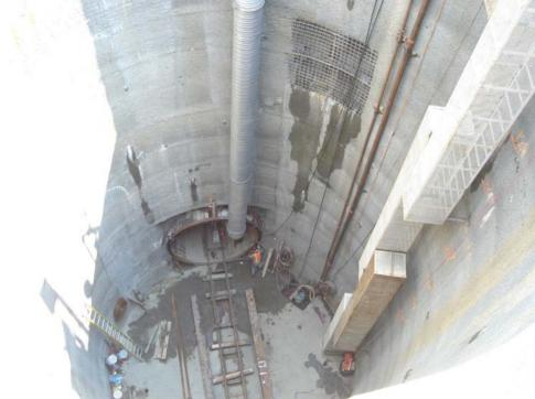
Components: •Steel Lattice Girders •Welded Wire Fabric •Shotcrete
