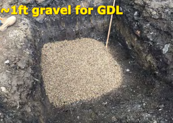
Installing gas probes
