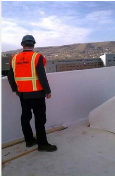
2015: Best PtD ELIMINATES fall hazard (Parapet at a different facility)*
