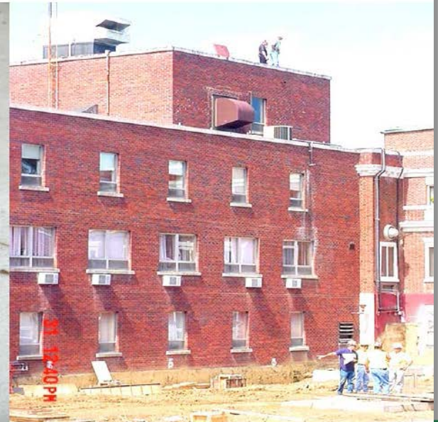
1940/50: NO fall protection & later HVAC placed near edge (old hospital wing)*
